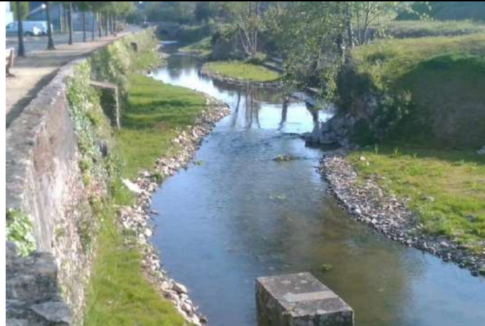
Figure 10 : Station ESTIMHAB (vue générale) UG5 (Fish-Pass)
